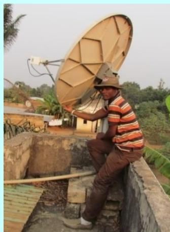
Early in 2015, the arms of the satellite communication system in Bukavu diocese were replaced and an improvement in the signal ensured the quality of the connection. This was followed by trouble-shooting and resetting of the satellite direction towards East Africa with the sole purpose of improving the service, this time in the diocese of the two Kasais which had been without a connection for almost a month in June 2015. A change in the VSAT antenna
